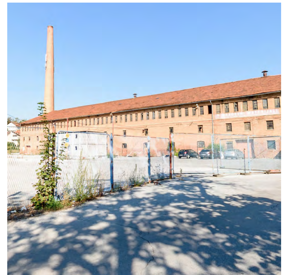
EXISTING SITUATION (GOGGLE STREETVIEW, 2019)
