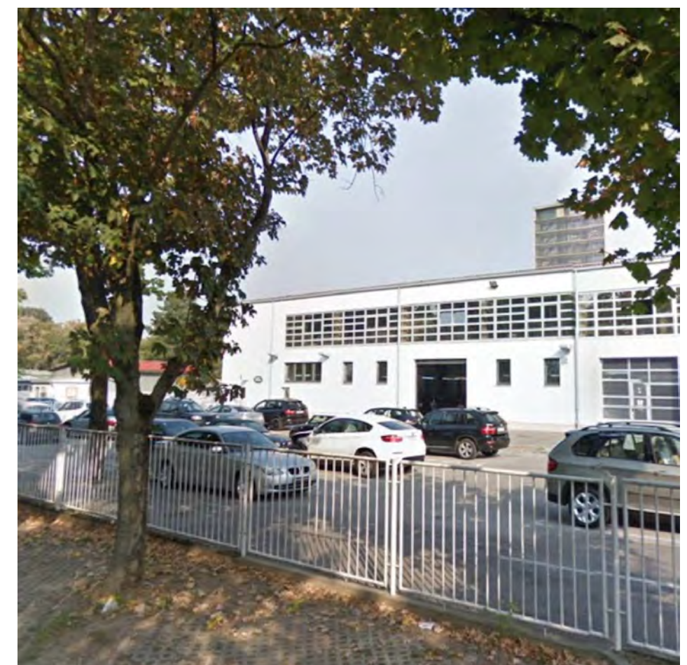
EXISTING SITUATION (GOGGLE STREETVIEW, 2011)
