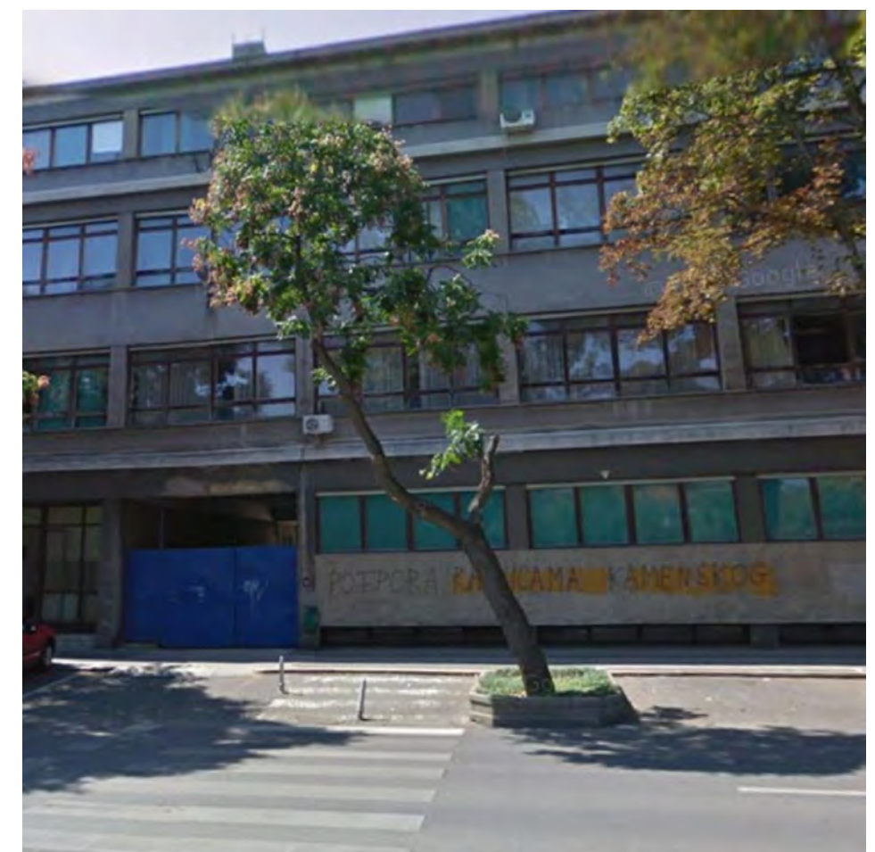
EXISTING SITUATION (GOGGLE STREETVIEW, 2011)
