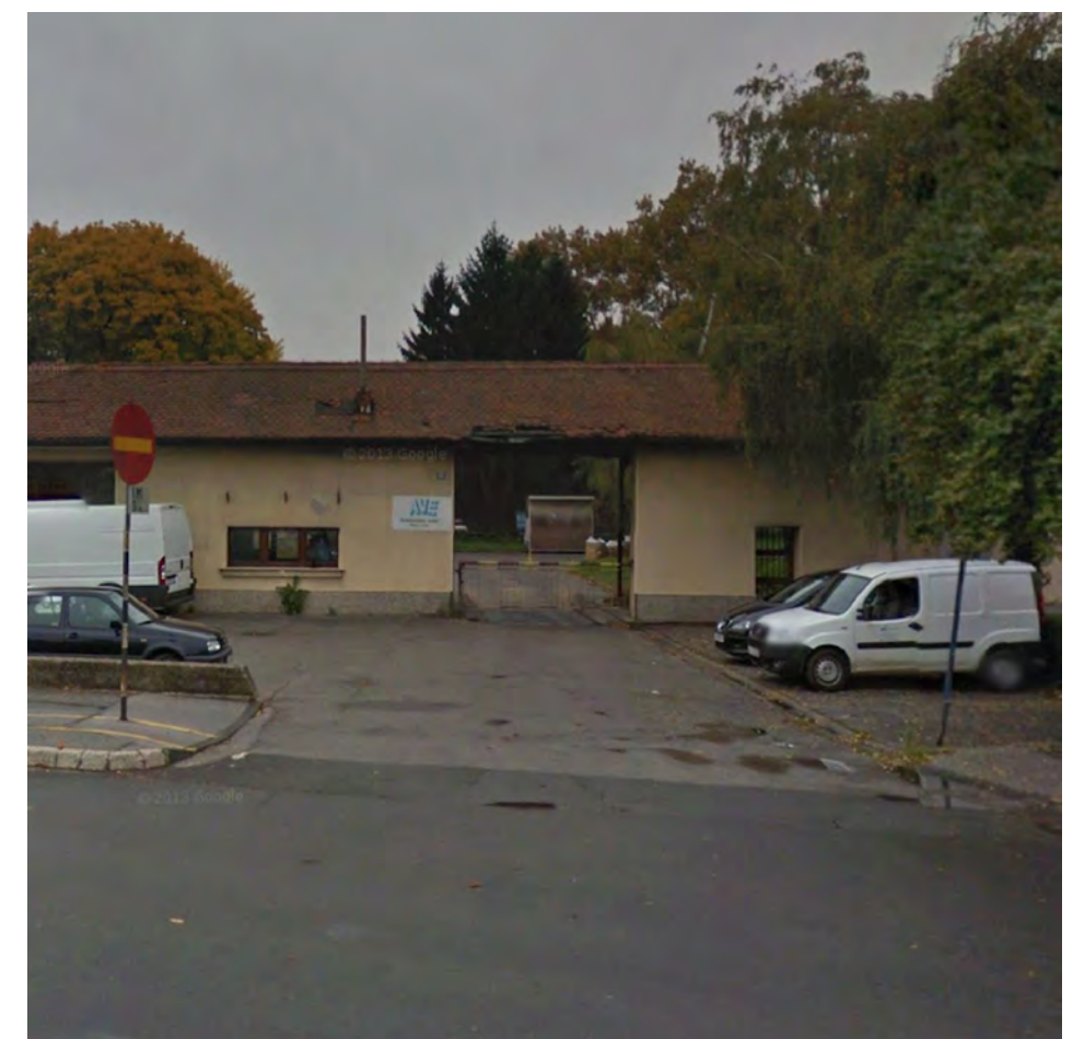
EXISTING SITUATION (GOGGLE STREETVIEW, 2011)
