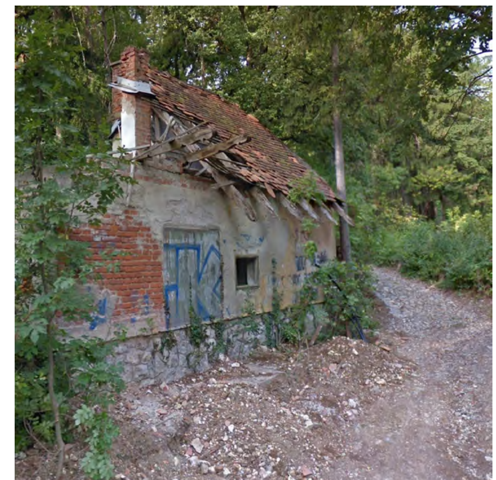
EXISTING SITUATION (GOGGLE STREETVIEW, 2011)
