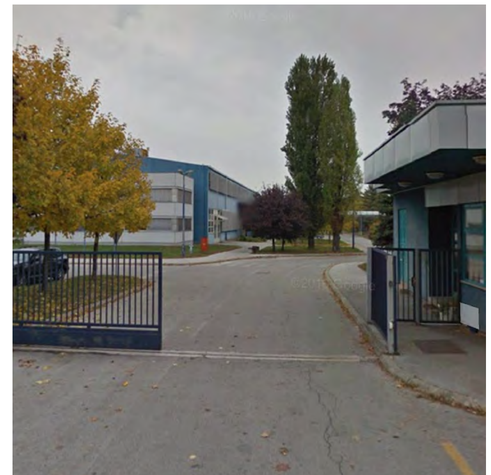
EXISTING SITUATION (GOGGLE STREETVIEW, 2011)
