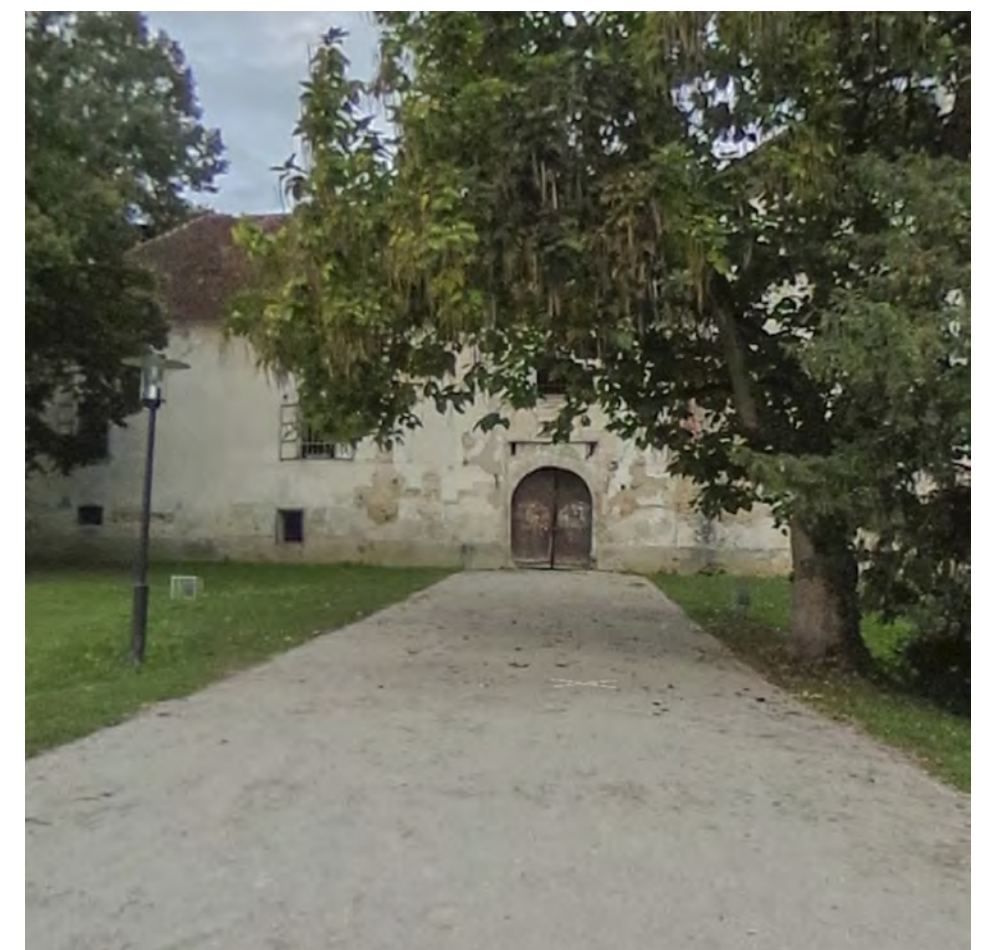
EXISTING SITUATION (GOGGLE STREETVIEW, 2011)
