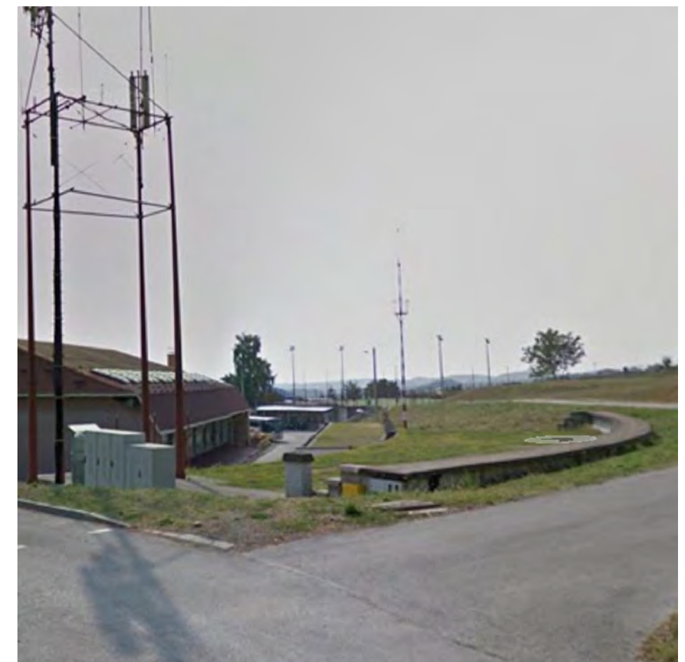
EXISTING SITUATION (GOGGLE STREETVIEW, 2011)
