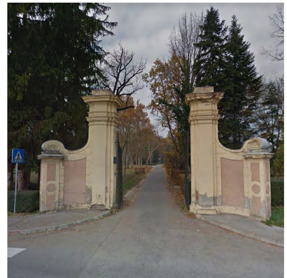
EXISTING SITUATION (GOGGLE STREETVIEW, 2011)
