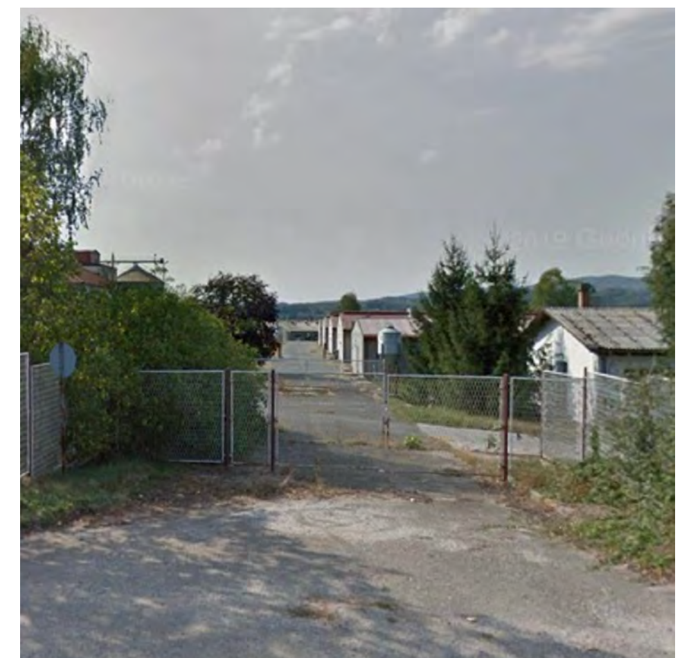
EXISTING SITUATION (GOGGLE STREETVIEW, 2011)
