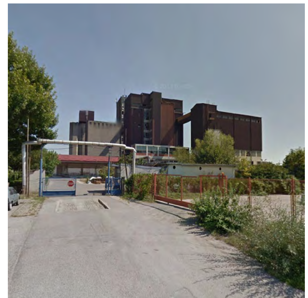
EXISTING SITUATION (GOGGLE STREETVIEW, 2011)
