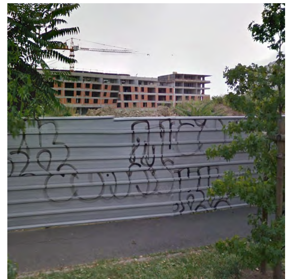
EXISTING SITUATION (GOGGLE STREETVIEW, 2011)
