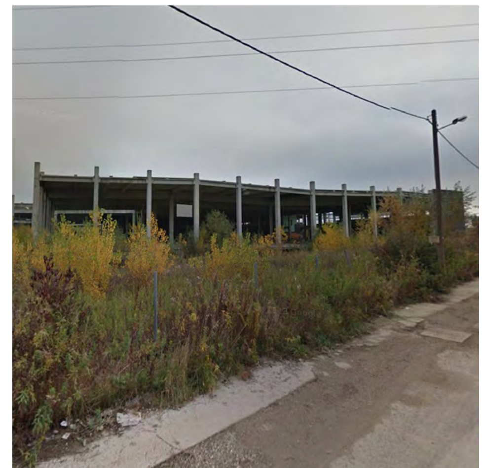
EXISTING SITUATION (GOGGLE STREETVIEW, 2011)
