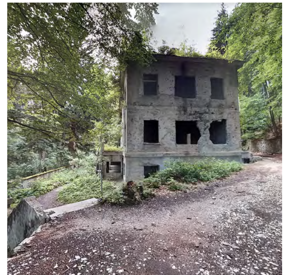
EXISTING SITUATION (GOGGLE STREETVIEW, 2013)
