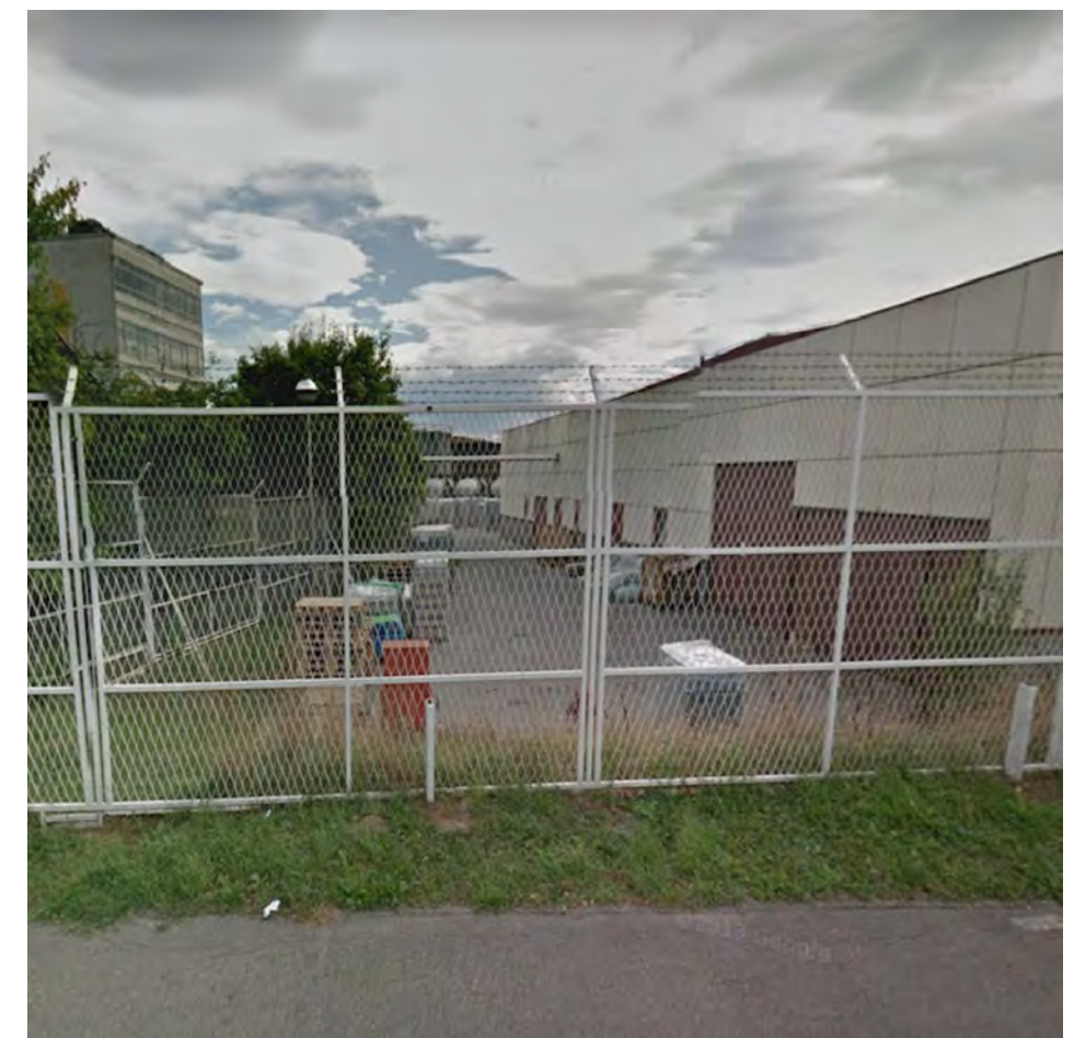
EXISTING SITUATION (GOGGLE STREETVIEW, 2012)
