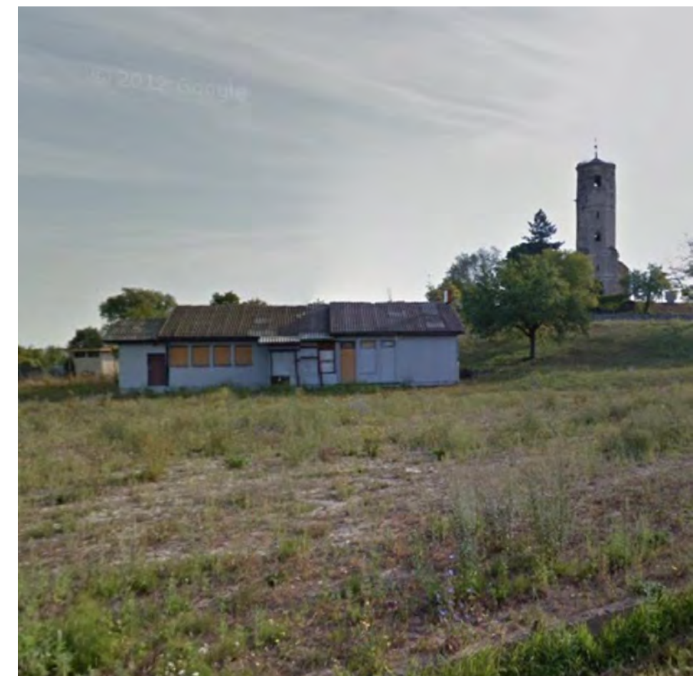
EXISTING SITUATION (GOGGLE STREETVIEW, 2011)
