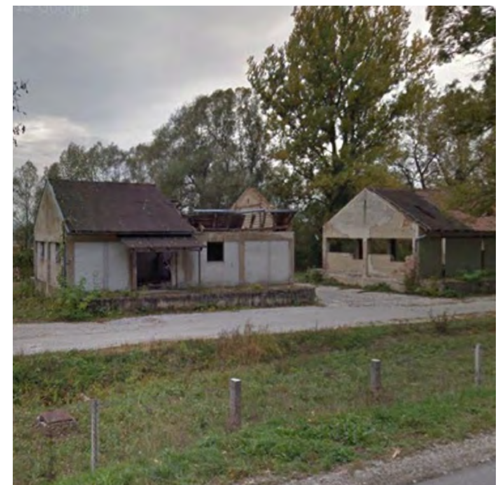
EXISTING SITUATION (GOGGLE STREETVIEW, 2011)
