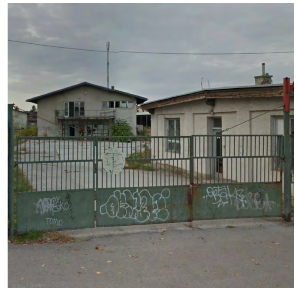
EXISTING SITUATION (GOGGLE STREETVIEW, 2011)
