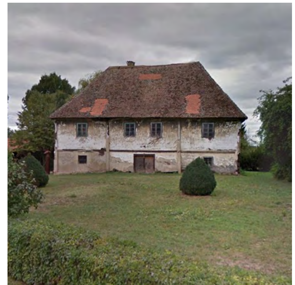
EXISTING SITUATION (GOGGLE STREETVIEW, 2011)
