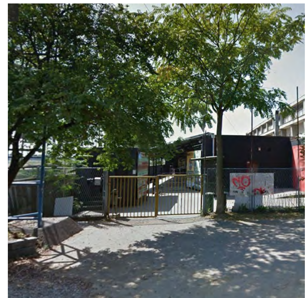
EXISTING SITUATION (GOGGLE STREETVIEW, 2011)
