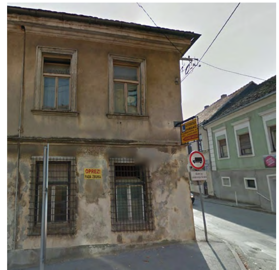
EXISTING SITUATION (GOGGLE STREETVIEW, 2011)
