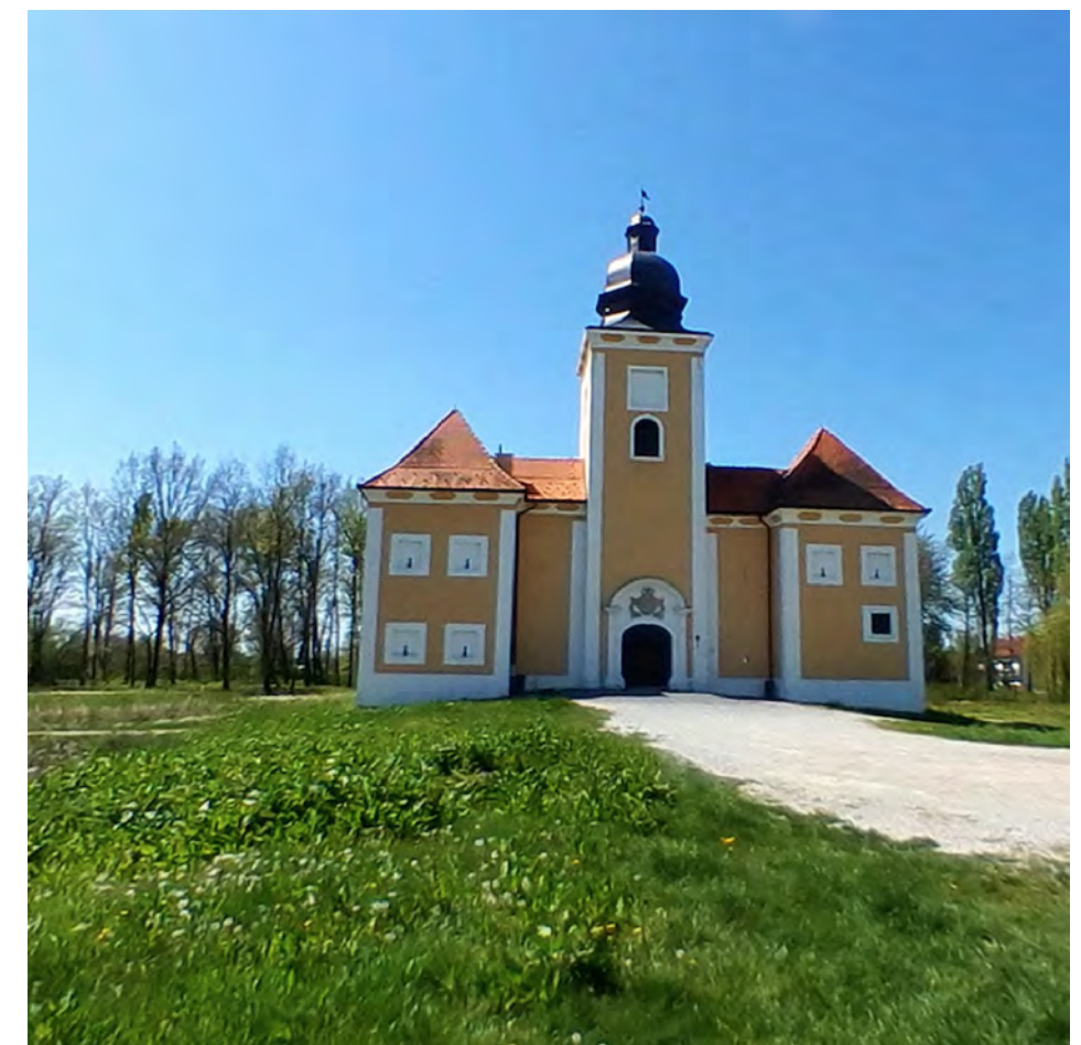
EXISTING SITUATION (GOGGLE STREETVIEW, 2011)
