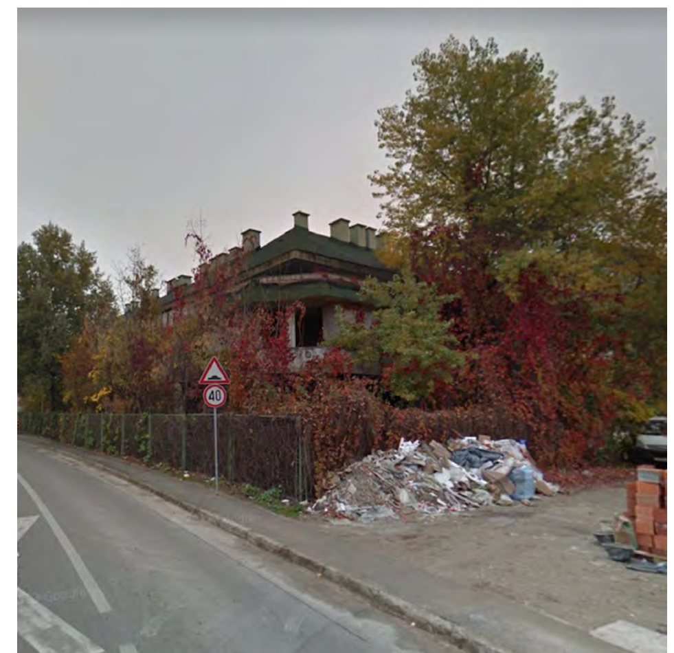
EXISTING SITUATION (GOGGLE STREETVIEW, 2011)
