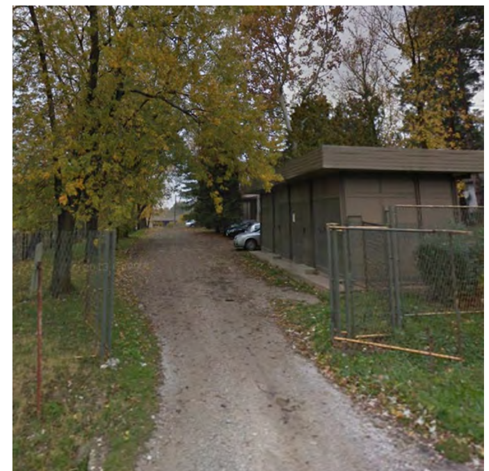
EXISTING SITUATION (GOGGLE STREETVIEW, 2011)
