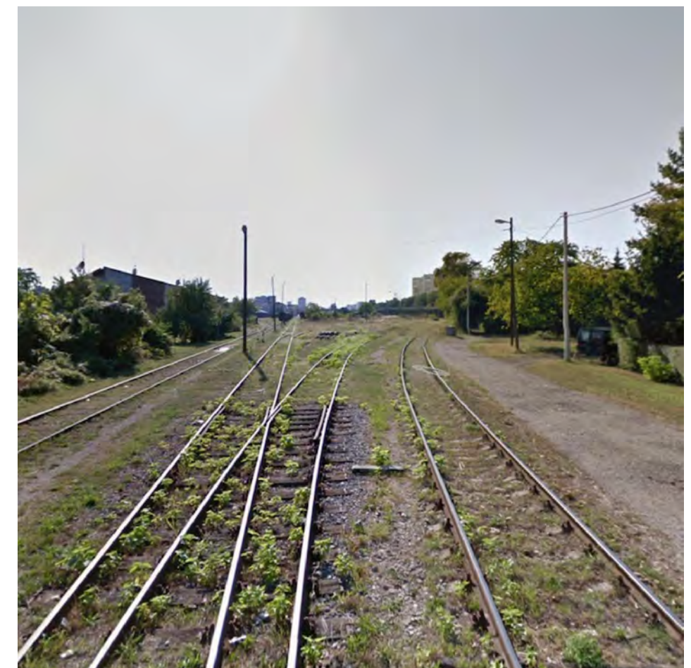
EXISTING SITUATION (GOGGLE STREETVIEW, 2011)
