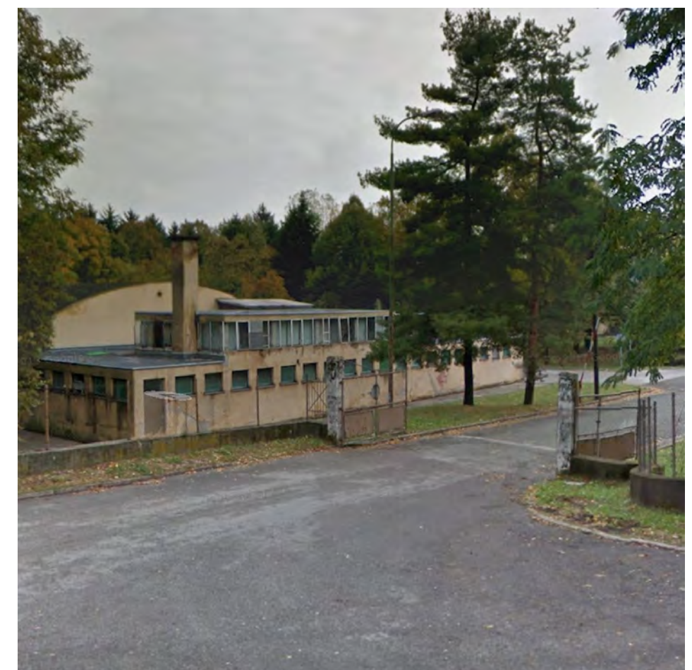
EXISTING SITUATION (GOGGLE STREETVIEW, 2011)
