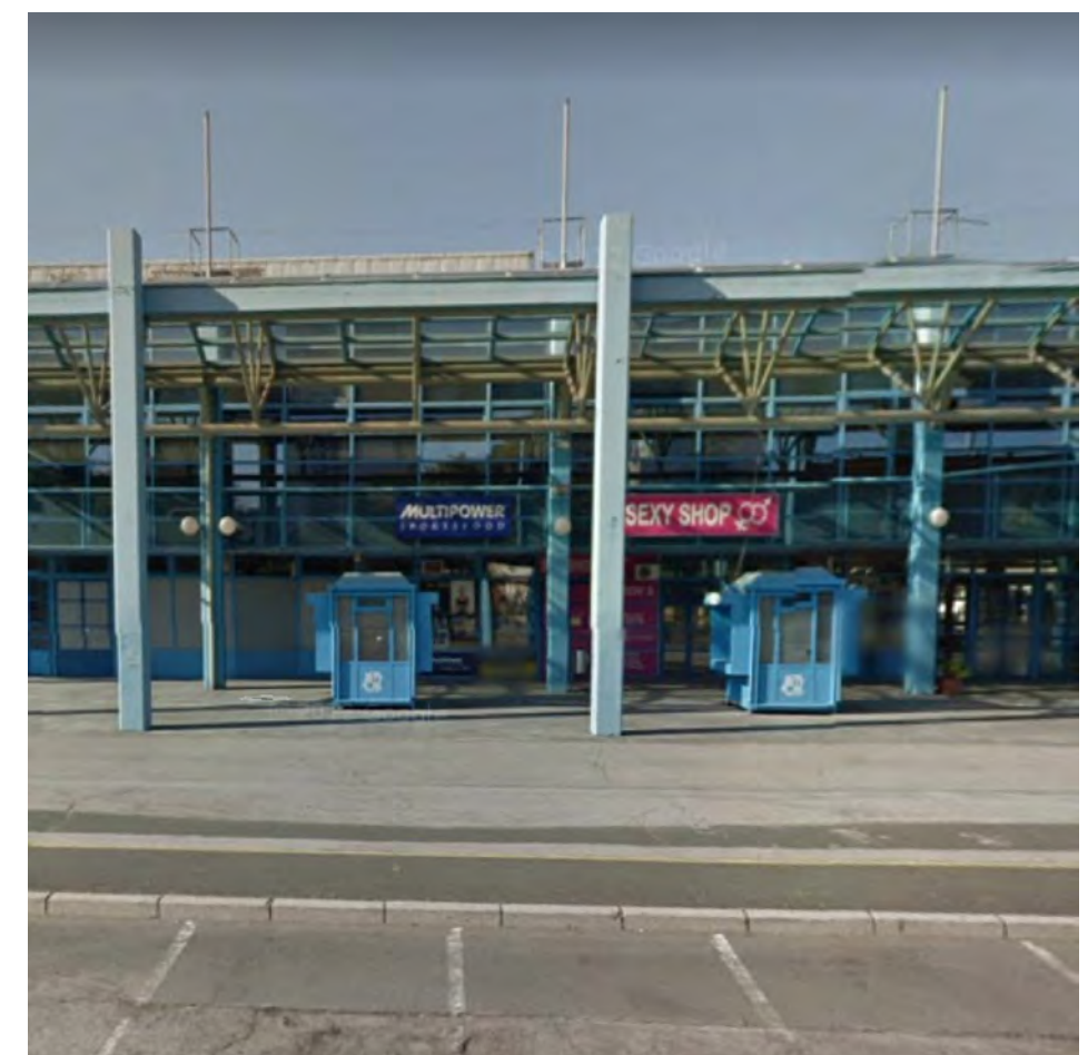
EXISTING SITUATION (GOGGLE STREETVIEW, 2011)
