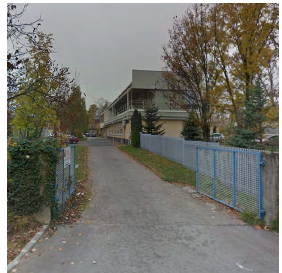
EXISTING SITUATION (GOGGLE STREETVIEW, 2011)
