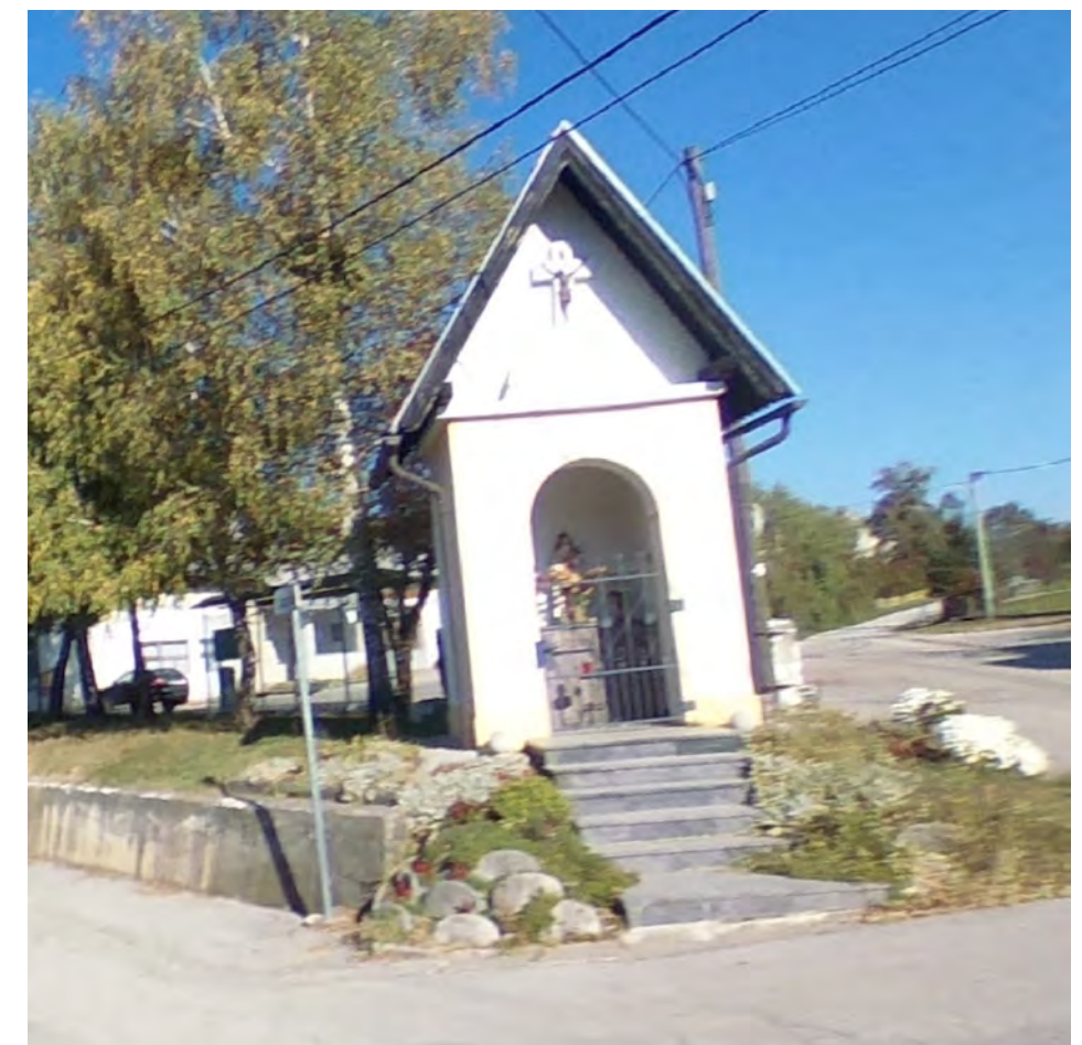
EXISTING SITUATION (GOGGLE STREETVIEW, 2011)
