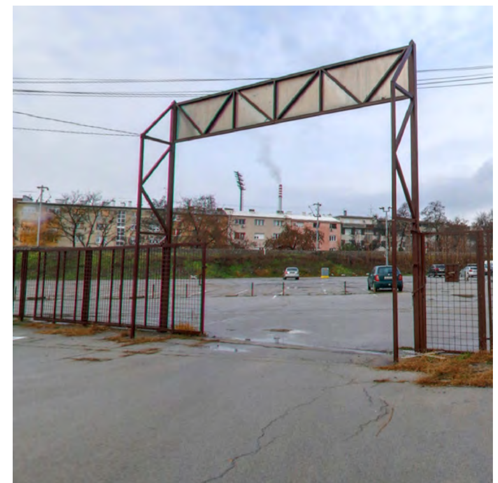
EXISTING SITUATION (GOGGLE STREETVIEW, 2011)
