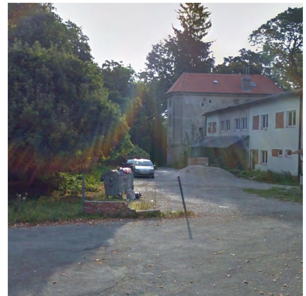
EXISTING SITUATION (GOGGLE STREETVIEW, 2011)
