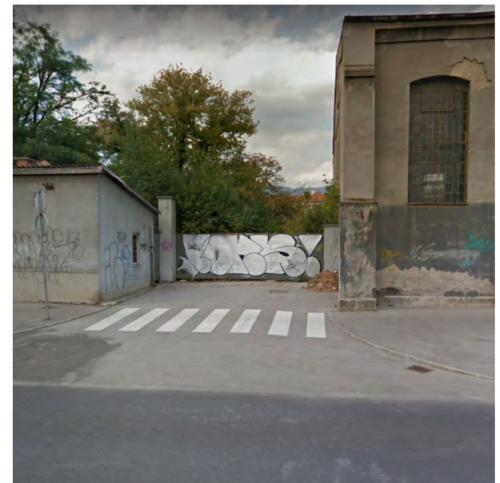
EXISTING SITUATION (GOGGLE STREETVIEW, 2012)
