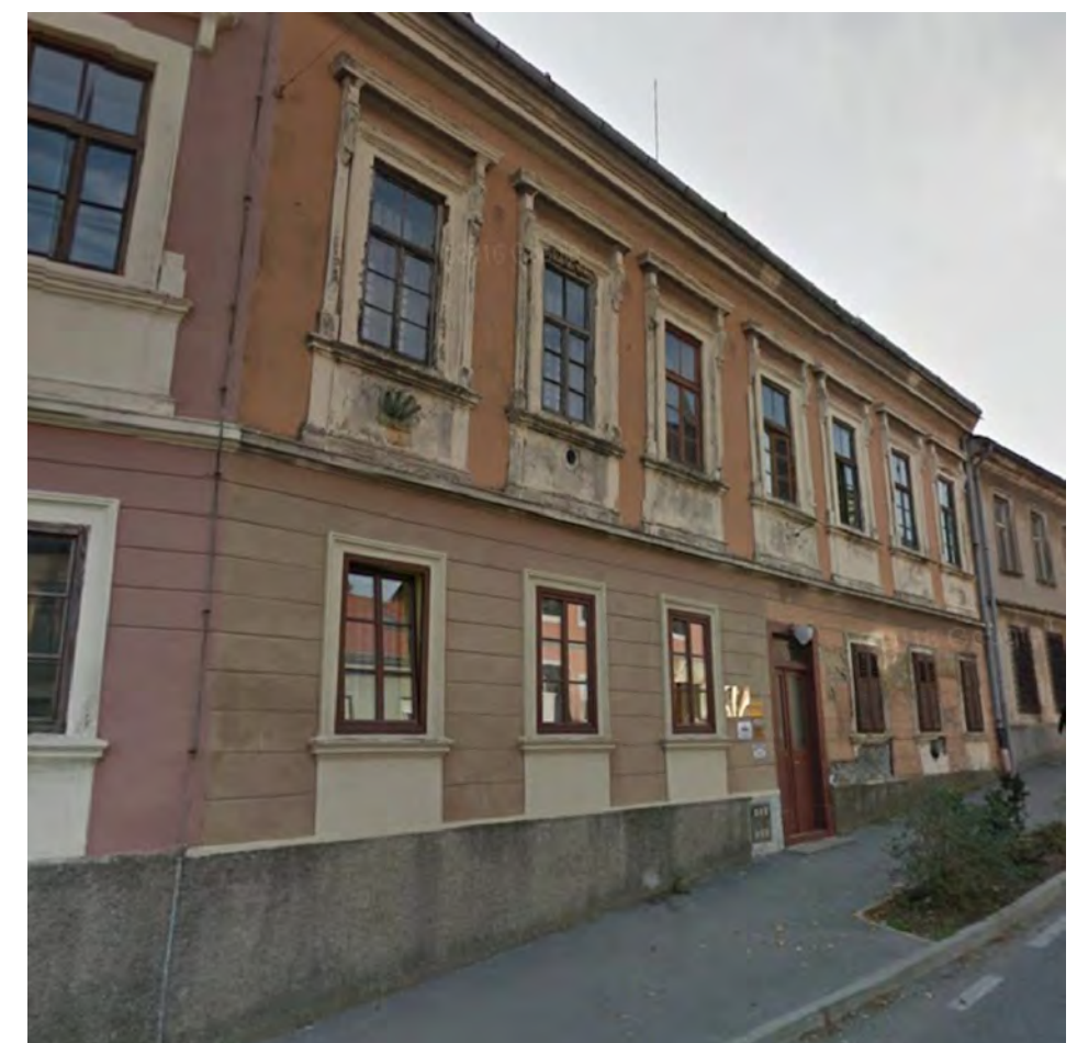
EXISTING SITUATION (GOGGLE STREETVIEW, 2011)
