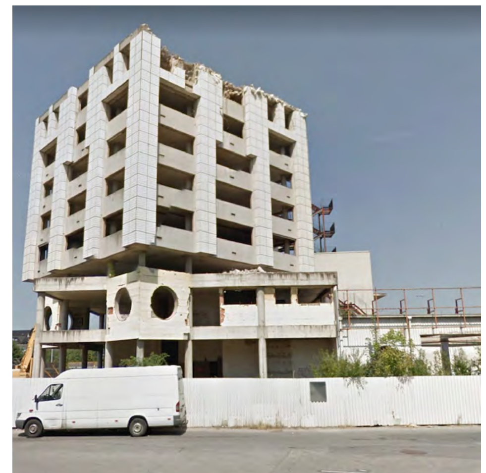
EXISTING SITUATION (GOGGLE STREETVIEW, 2011)
