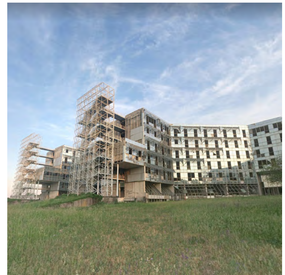
EXISTING SITUATION (GOGGLE STREETVIEW, 2018)
