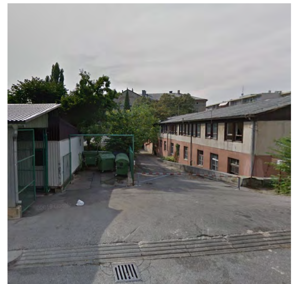
EXISTING SITUATION (GOGGLE STREETVIEW, 2011)
