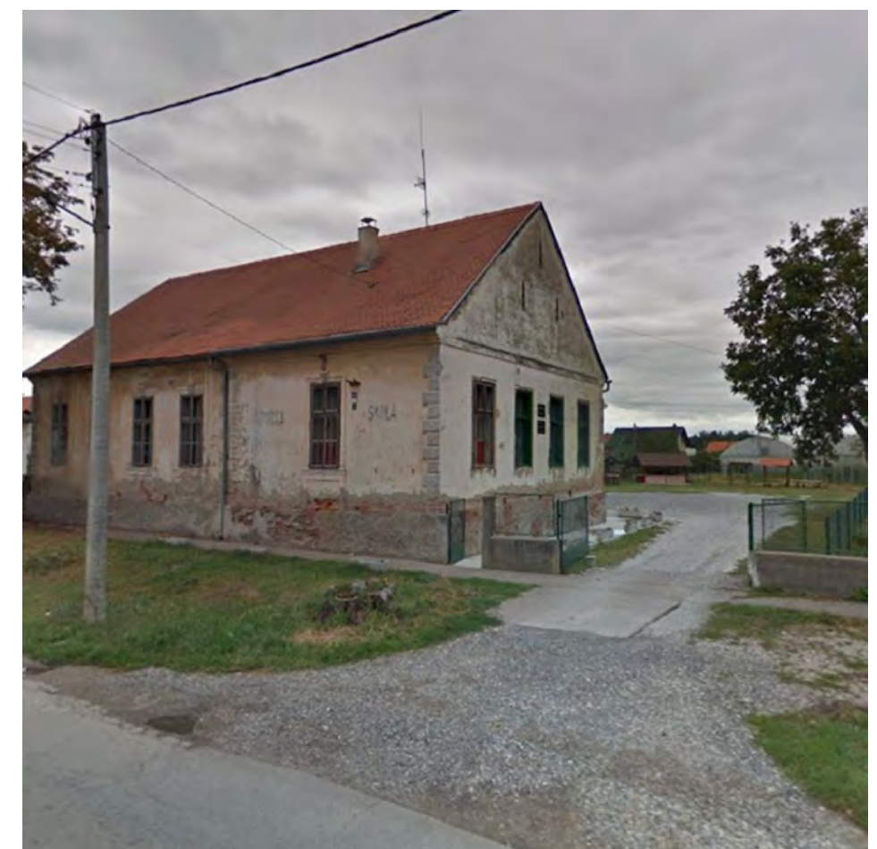
EXISTING SITUATION (GOGGLE STREETVIEW, 2011)
