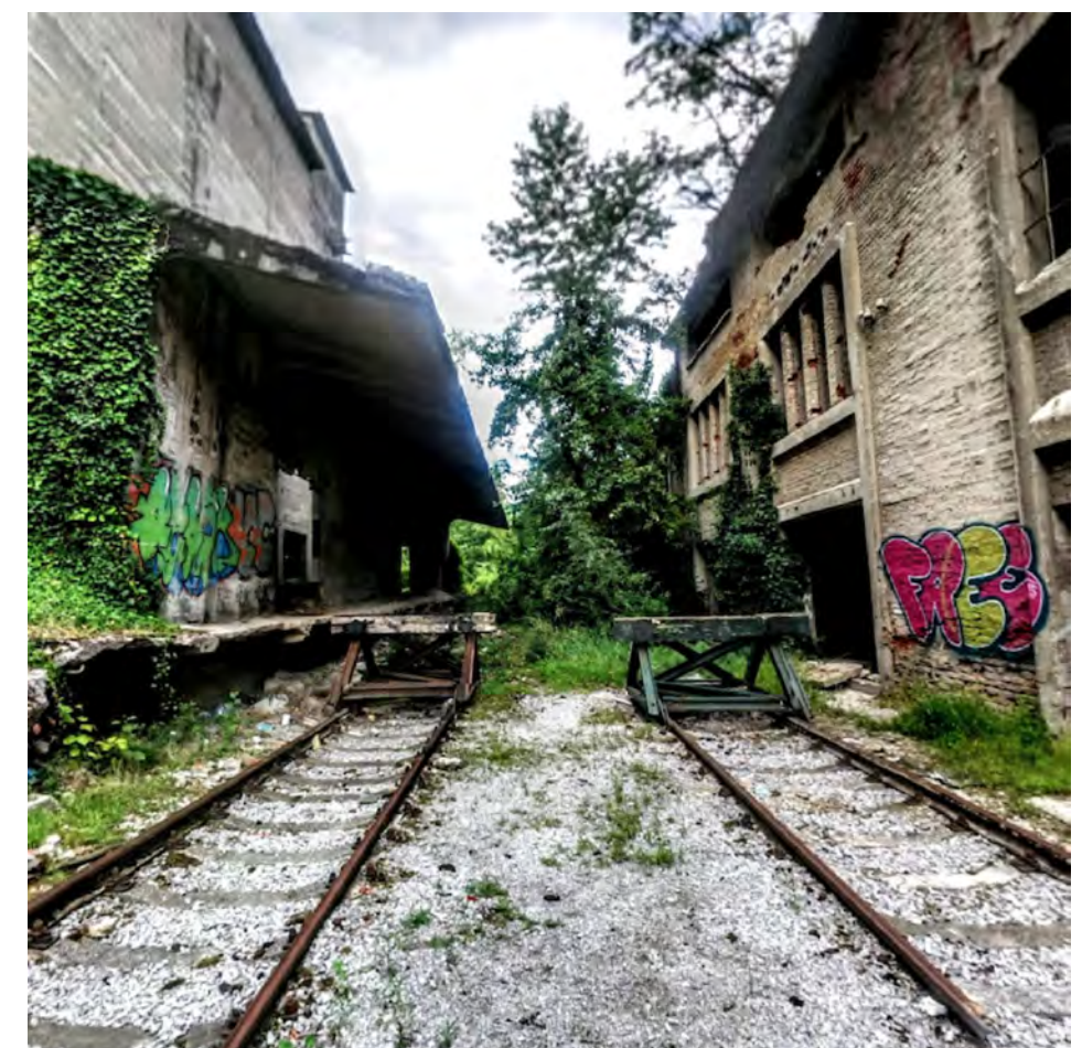
EXISTING SITUATION (GOGGLE STREETVIEW, 2016)
