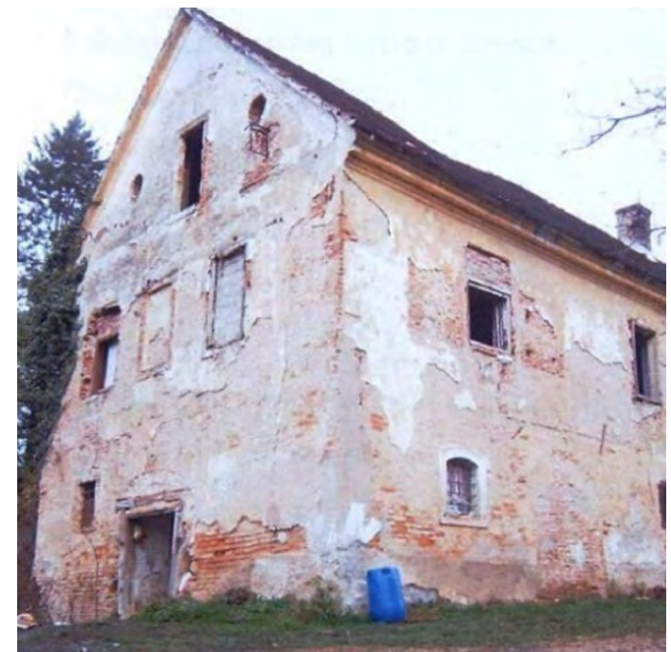
EXISTING SITUATION (GOGGLE STREETVIEW, 2011)
