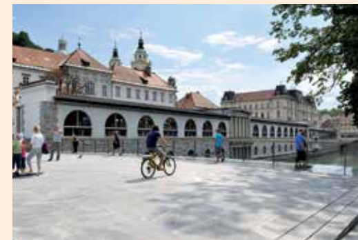
MESARSKI MOST – NOVI MOST PREKO RIJEKE LJUBLJANICE / MESARSKI MOST – A NEW BRIDGE ACROSS LJUBLJANICA RIVER
