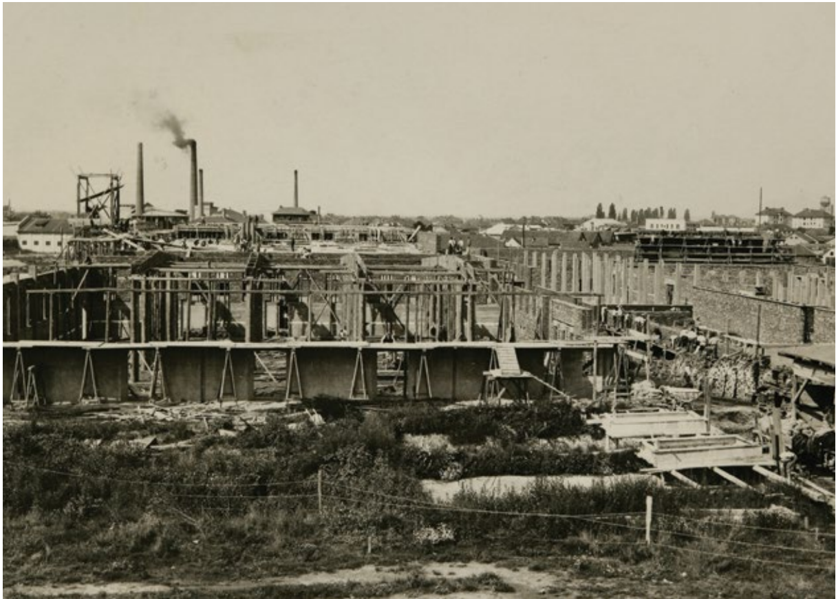
SLIKA 07 Izgradnja kompleksa Gradske klaonice i stočne tržnice u Zagrebu, oko 1929. / IMAGE 07 Construction of the City's slaughterhouse and cattle market in Zagreb, around 1929
