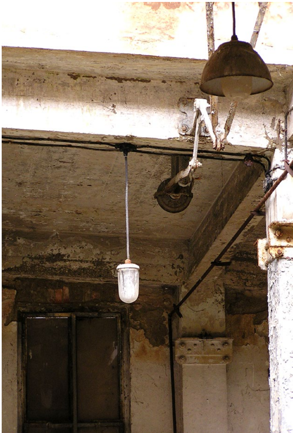
SLIKA 022 Detalj interijera klaoničke hale (rasvjetna tijela), 2014. / IMAGE 022 Detail of the interior of slaughtering halls (lighting fixtures), 2014
