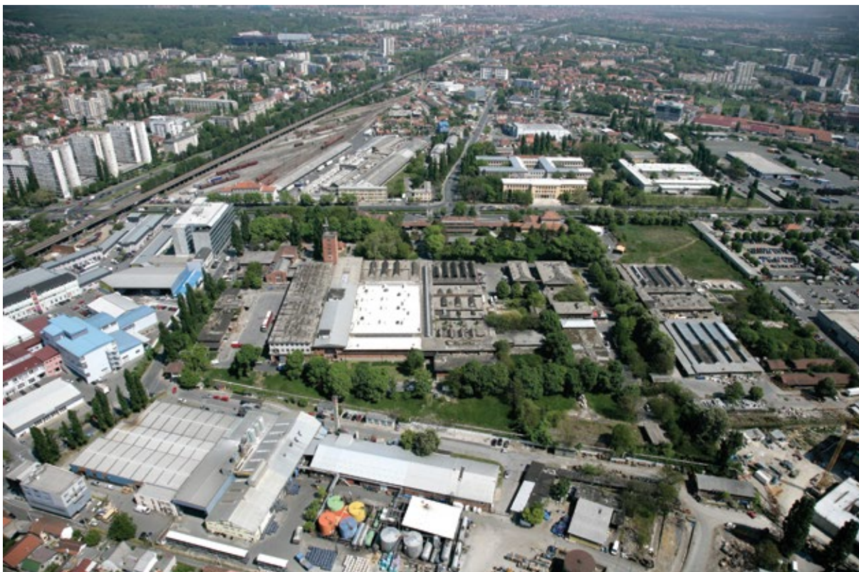
SLIKA 026 Pogled sa zapada na kompleks nekadašnje Gradske klaonice i stočne tržnice, 2007. / IMAGE 026 View from the west onto the complex of the former City's slaughterhouse and cattle market, 2007
