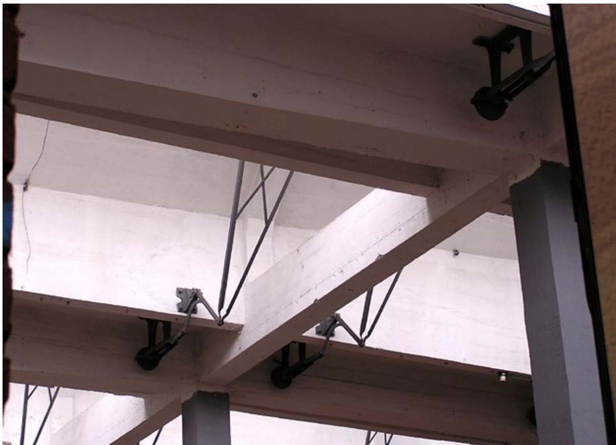
SLIKA 016 Detalj krovne konstrukcije u klaonici za krupnu stoku, 2014. / IMAGE 016 Detail of the roof structure on the cattle slaughterhouse, 2014
