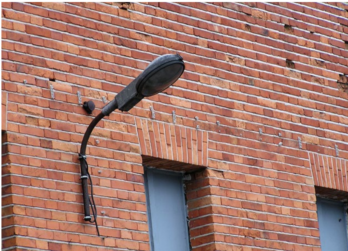
SLIKA 020 Detalj fasadne opne, 2014. / IMAGE 020 Detail of front layer, 2014
